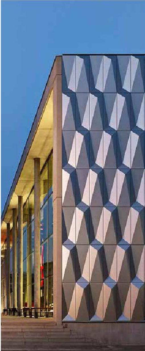
The negative space between the panels also gives the viewer an opportunity to observe their connections, interworking and functionality. The joints and connectivity built into the system do not go unnoticed. Parametric design allows for this type of intelligence to be built into the system, enabling the production and fabrication of these surfaces of complexity.
